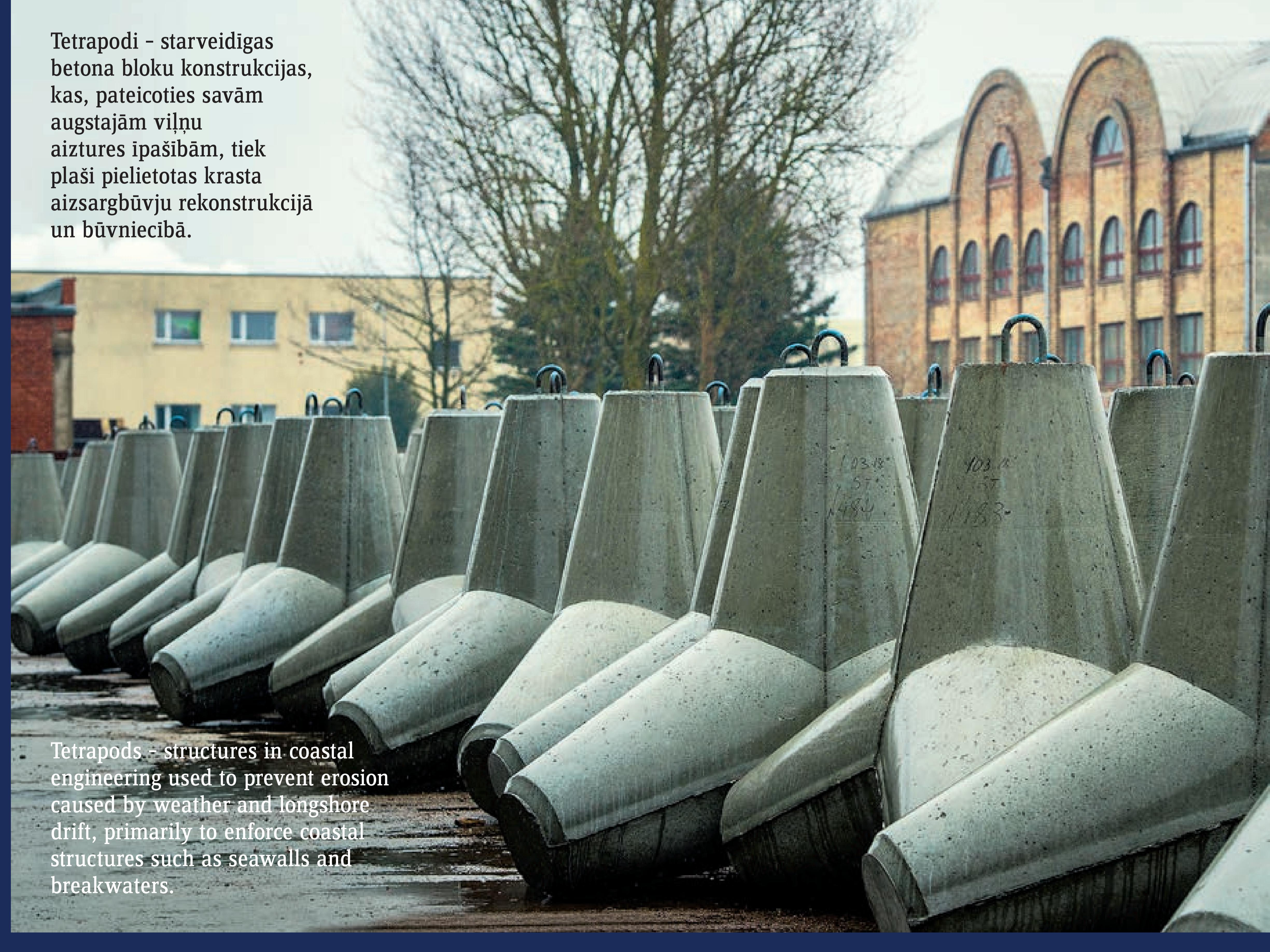
Tetrapods - structures in coastal engineering used to prevent erosion caused by weather and longshore drift, primarily to enforce coastal structures such as seawalls and breakwaters.
